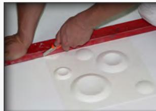
**Tip:** 3D Panels can be cut and abraded. Use these advantages to cut out the light switches or sockets and then abrade the cut for example. This must be done before you attach the panels.
