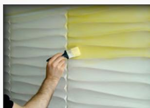
Before the painting procedure the 3D panels have to be primed with the special-primer by using a brush.
