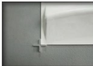
Press the 3D panels well to the prepared surface. Use tile crosses to ensure regular spaces between the 3D panels.
