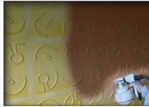
After the drying time of the special-primer (about 60 minutes), the 3D panels can be painted as desired. Common variants are wall paint, latex paint or varnish.
